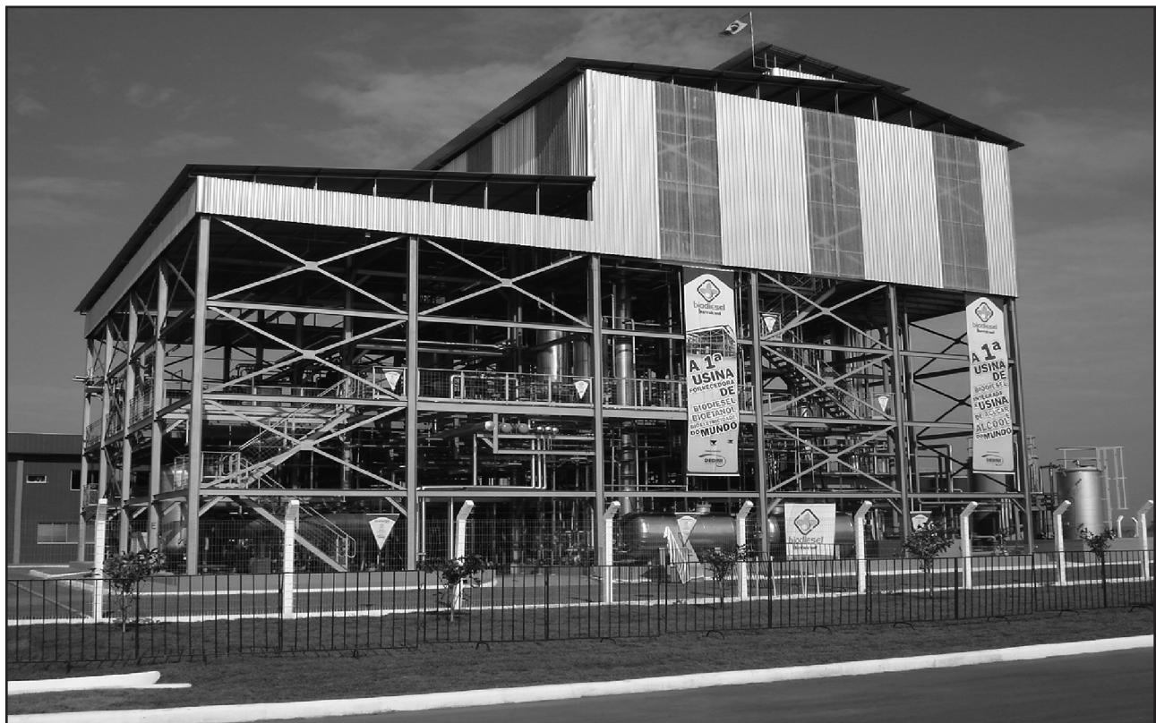
FIGURE 9 Barralcool Biodiesel Plant.
