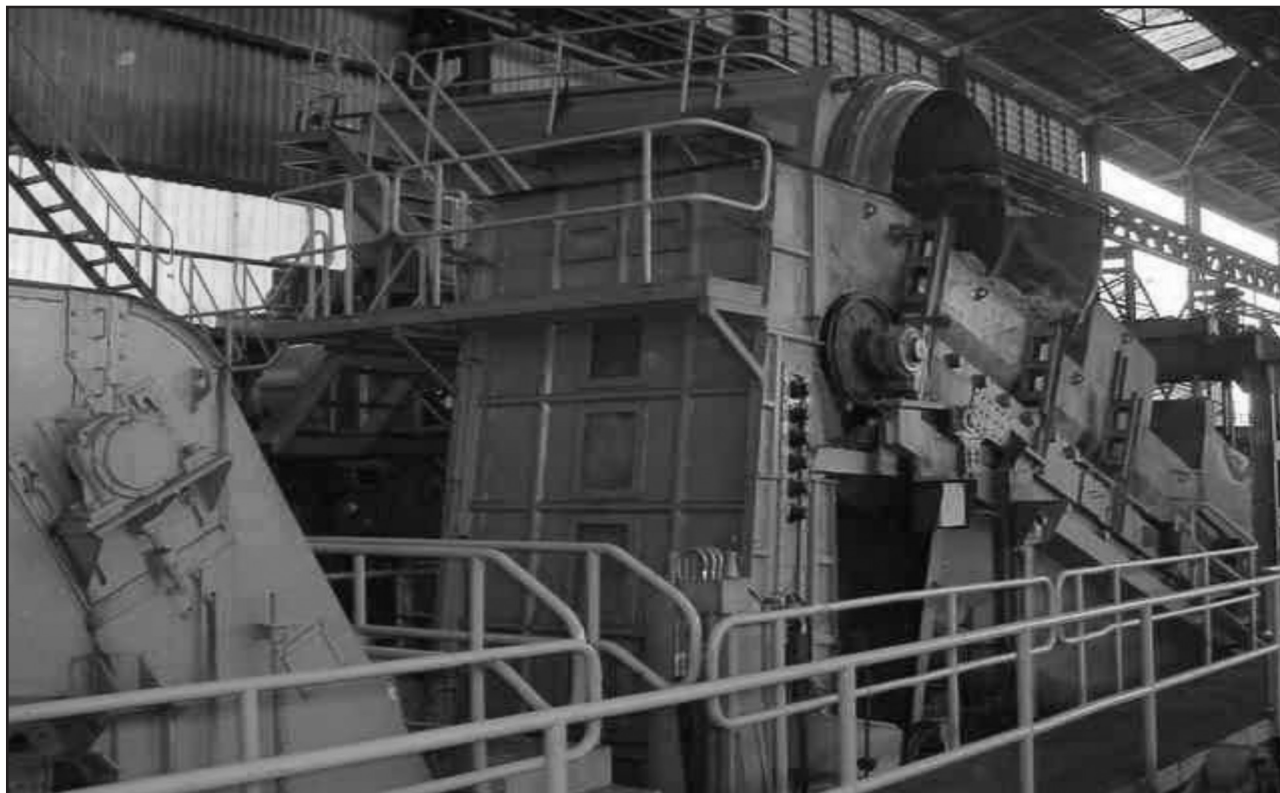
FIGURE 1 Donnelly chute installation at the first mill inlet.
