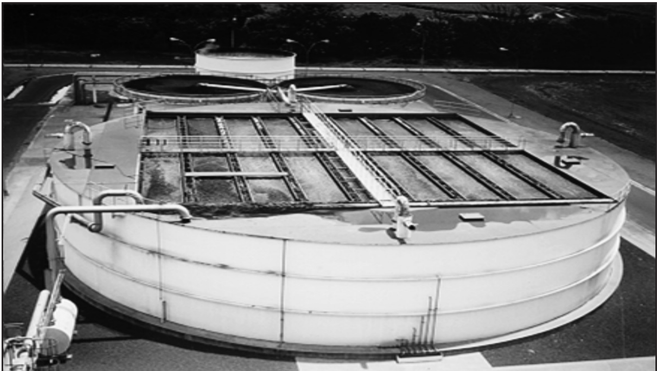
FIGURE 5 View of the bio-digester installed at Usina São Martinho.
