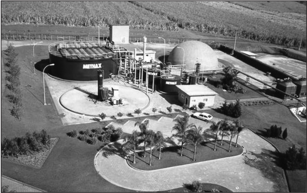
FIGURE 4 Picture of the Usina São João project showing the bio-digester and the gasholder.
